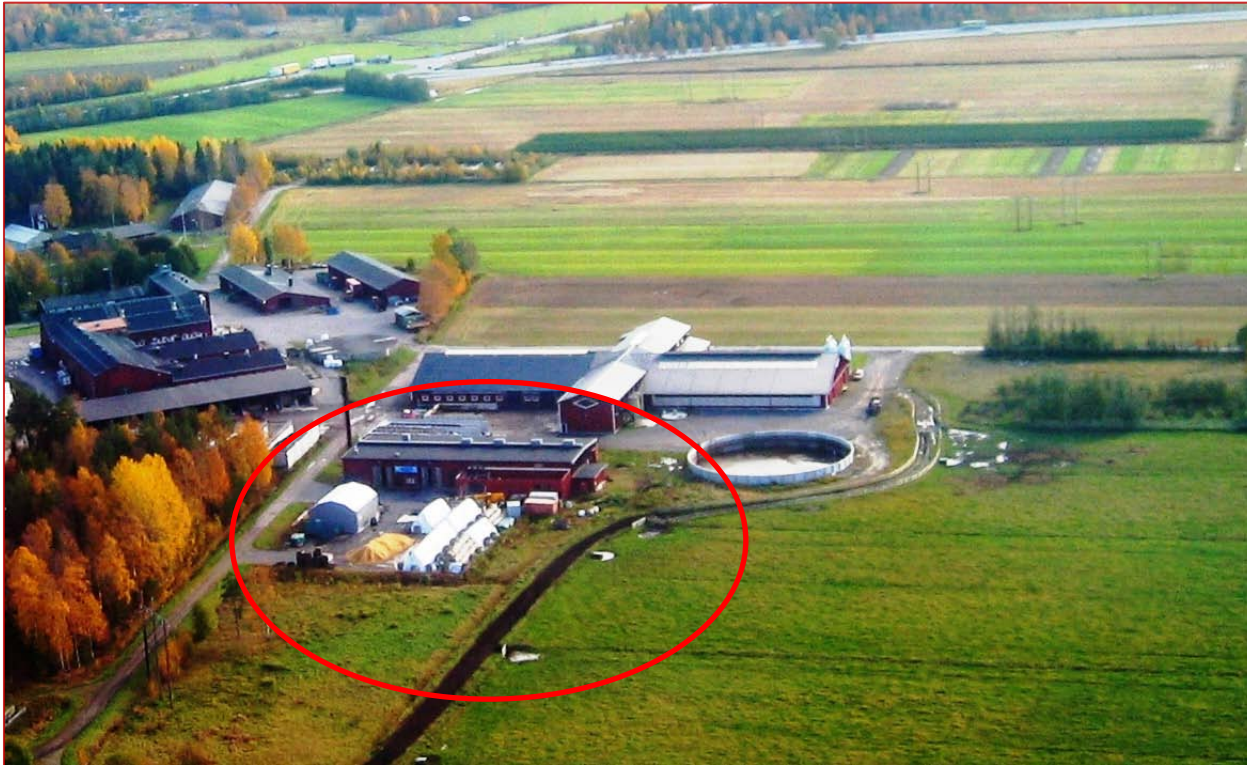
Research pilot plant BTC, Umeå
