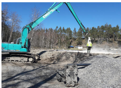
Pilot scale experiments of mixing fly ash from Naantali multifuel power plant and other industrial by-streams to stabilize earth in Naantali Housing Fair 2022 area
